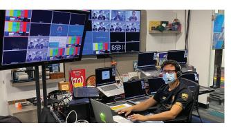
BROACAST FACILITIES: 3 production switchers, 256x256 3G Router, Haivision SRT encoding for transmission and remote contributors, 8 camera package, 8 Zoom stations, Ventuz real-time graphics system, 16 Channels of embeddable audio for multi-language support, 12 Channels of record decks, including support for archival ProRes and real-time MP4 availability
